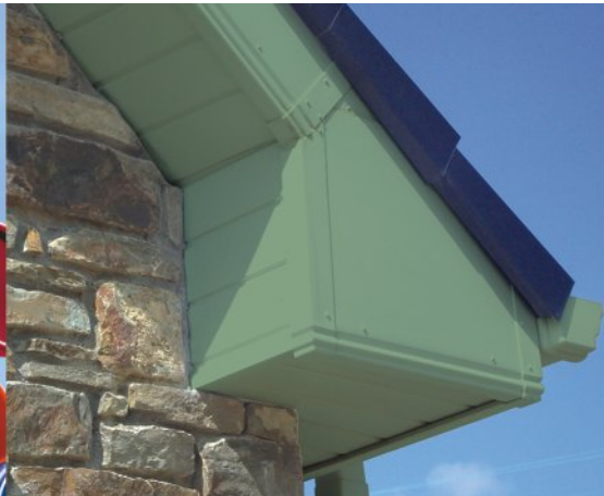
SOFFITS AND SIDINGS
