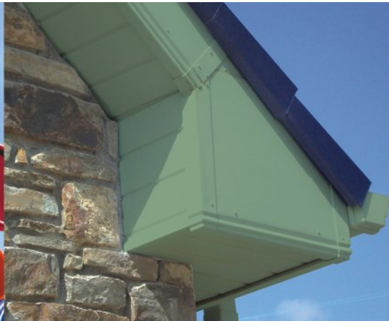
SOFFITS AND SIDINGS
